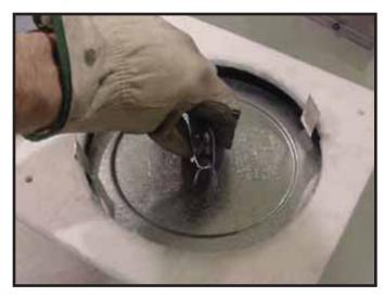
**Figure 9.4** Fold the center parts of the retaining band up and use to remove the seal cap.
